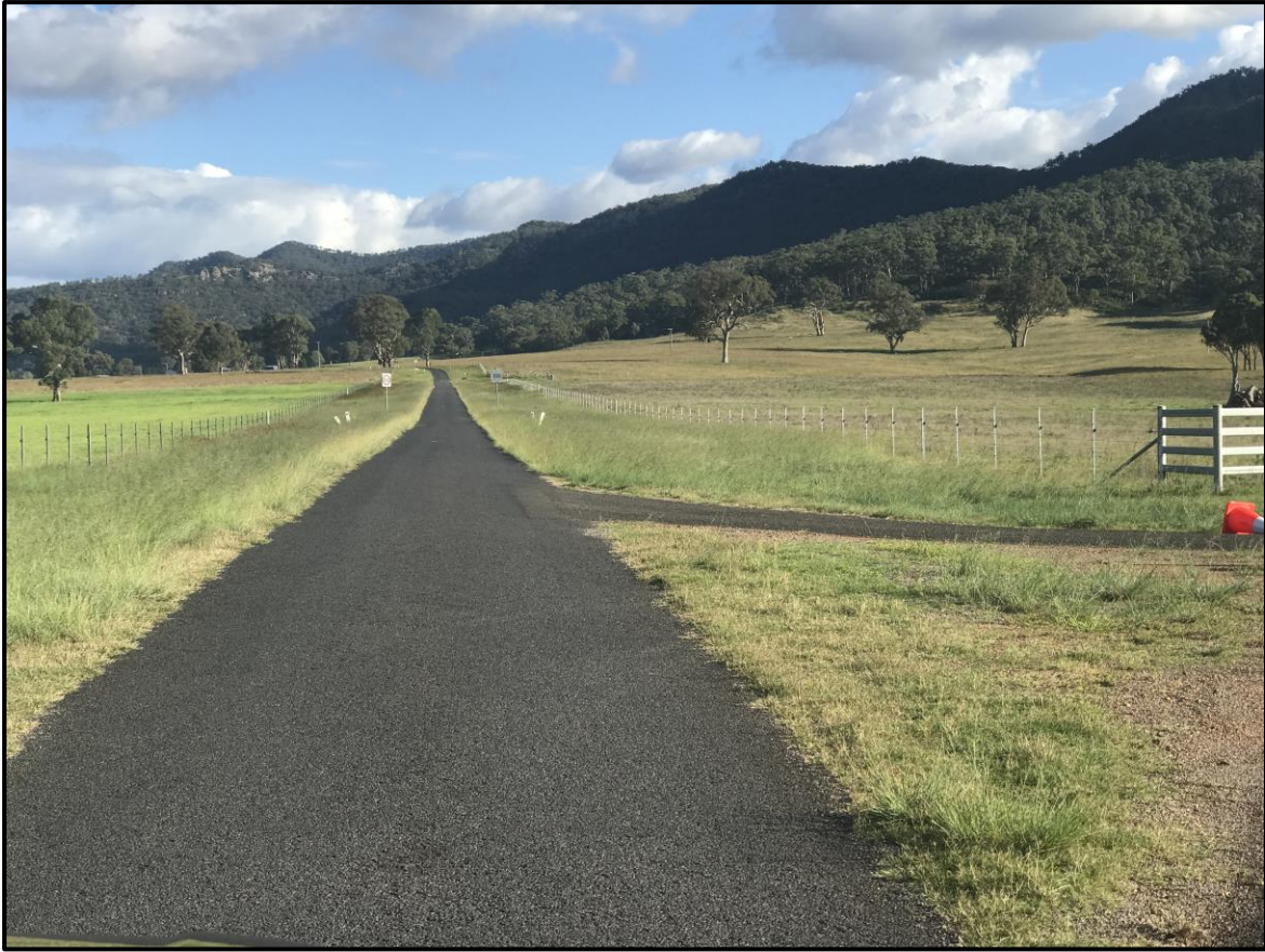
Photo 5 – Section of Martindale Road to south of the bridge crossing over Martin Dale creek, showing straight alignment and clear advanced visibility for drivers travelling in both directions.
