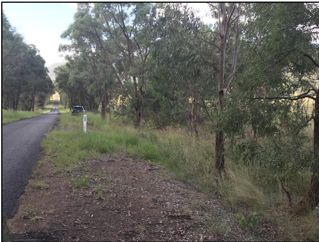
Photo 2 – View north along Martindale Road to immediate south of site access (car parked in access). Removal of the trees / vegetation to the left will highlight the presence of the access and improved visibility.
