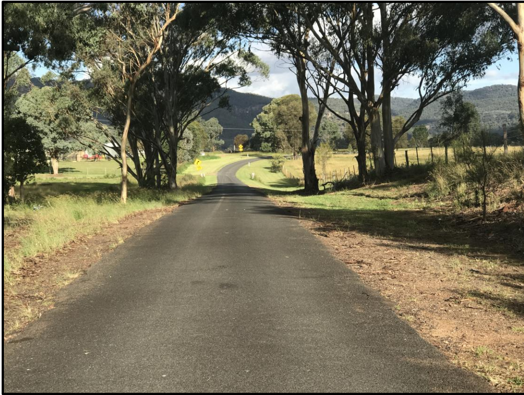
Photo 1 – nominated location (chainage 2100) for formal sealing of shoulders to allow for passing vehicles
